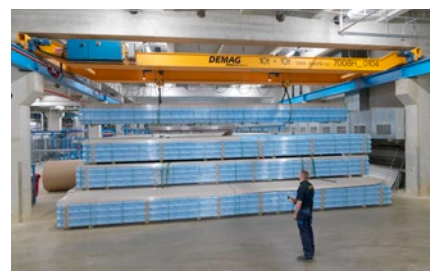
Overhead travelling crane for handling cores
